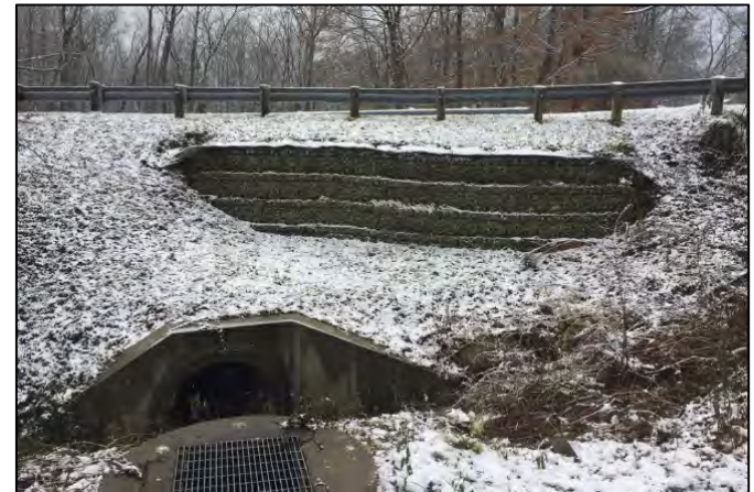
Slumping gabions next to road
