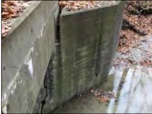
Cracked bridge abutment
