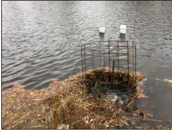
Existing outlet structure that could potentially be optimized to reduce downstream erosion.
