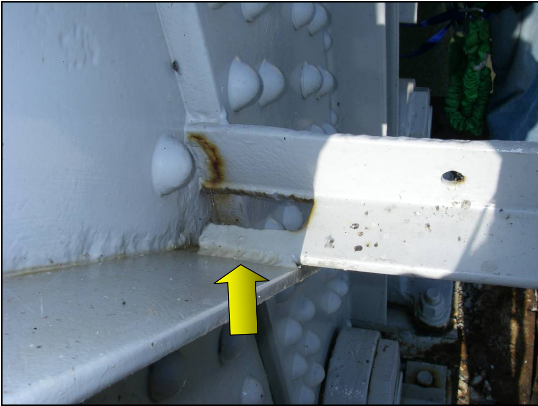
Figure 5- Welded brackets for stream monitoring equipment in spans 4 and 5
