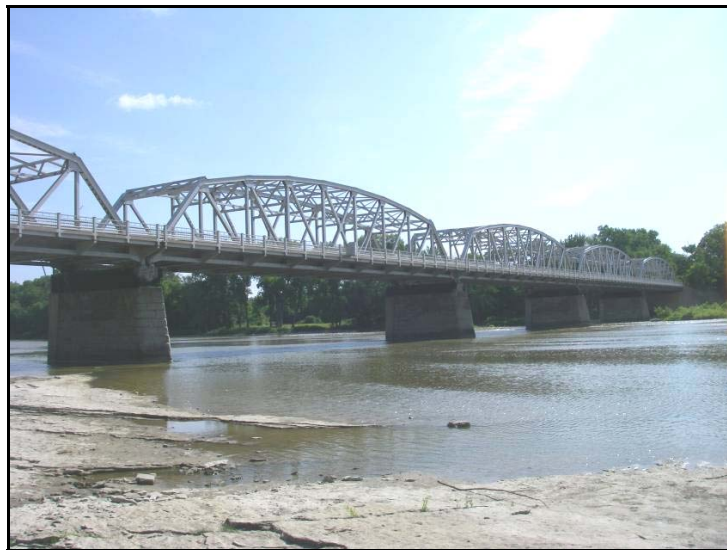
Figure 1 - Woo-64-1203 – Elevation looking northeast
